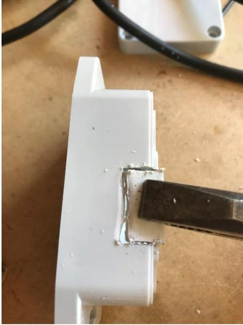
After taking the lid off the junction box, I cut (using a side cutter) slots down one side to create where the power cable (to the C64) will exit the box. Here I am snapping off the section between the two cuts I made.
